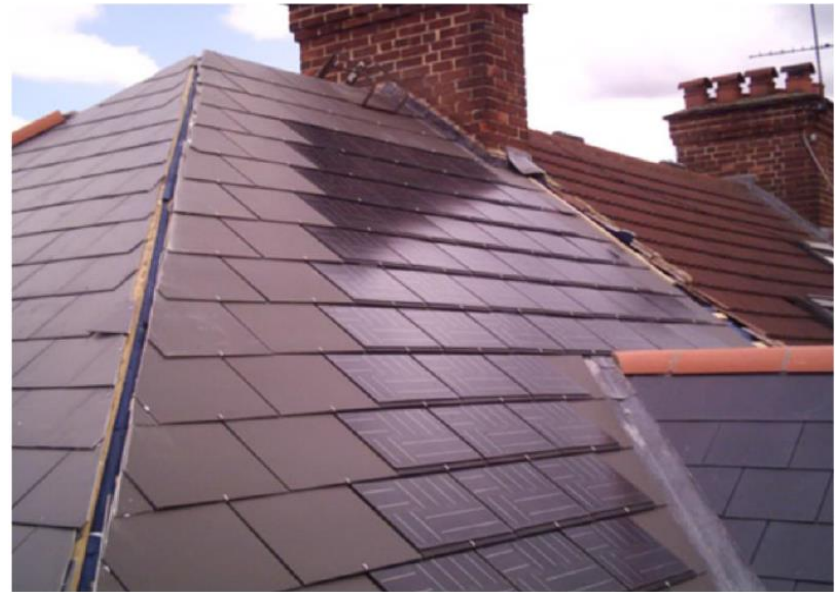
BIPV tiles on a roof
