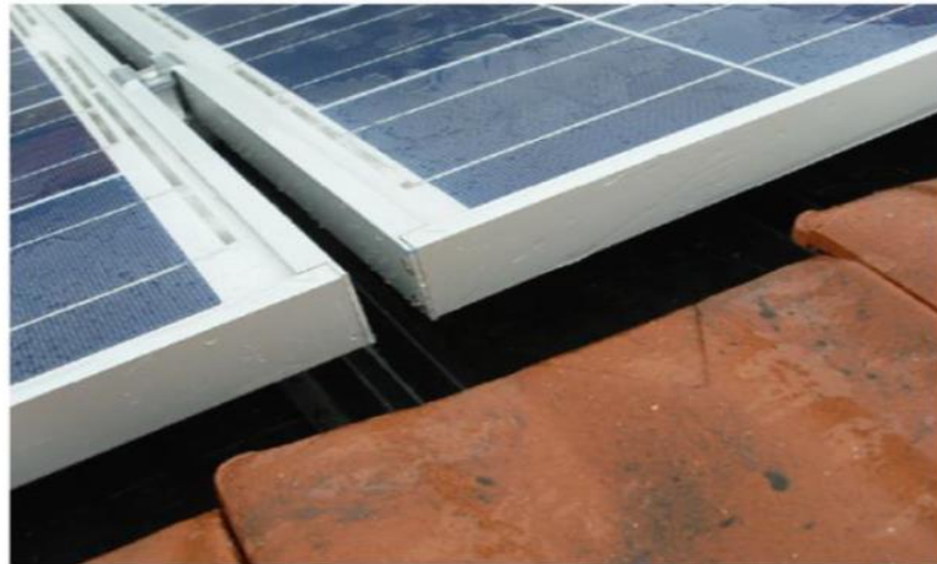
BAPV module on tile roof
